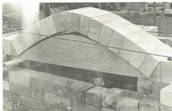
The firemouths and bases of bagwalls.
