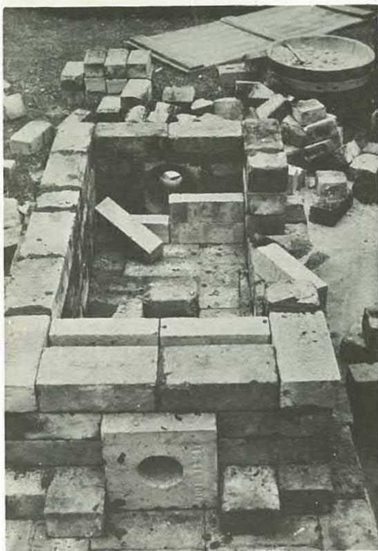
The floor, showing flue.
