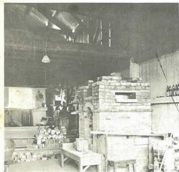
KILN UNDER CONSTRUCTION
