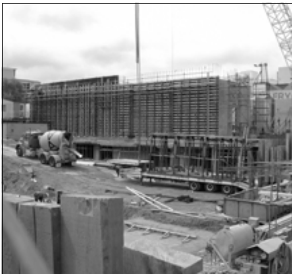
Another concrete truck arrives on site.
